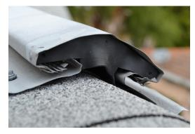
Metal ridge vents are capped with a rubber boot which allows Bats, Rats, Mice, and other rodents to push their way past the rubber boot and directly Into the attic.
