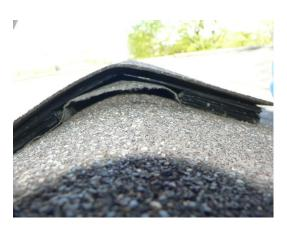
Plastic ridge vent without end cap. Opening allows Bats, Mice, Bees, Wasps and small rodents direct access to the attic
