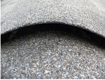
Overhang can be 2-3 inches longer than vent
