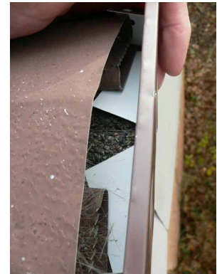
On the metal ridge vents, slide EndCap™ between roof shingle and metal ridge vent. Push EndCap™ tight against ridge vent, bend tabs tight against ridge vent and secure with screws provided.
