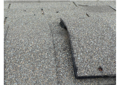
Shingle trimmed flush with end of ridge vent
