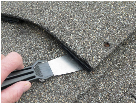
Use Putty Knife or straight blade and slide between roof shingle and the ridge vent so EndCap™ will slide between them easily.
