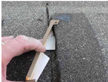
Slide one end of the EndCap™ in above the roof shingle and under the Ridge vent. Work the rest of the EndCap™ under the other side of ridge vent and push it up tight against the ridge vent. Bend tabs down tight and secure with nails provided.
