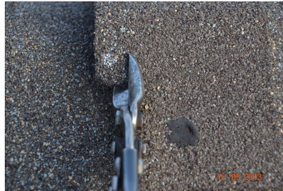
Trim overhang flush to end of ridge vent
